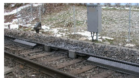
Rail flanks lubrication
