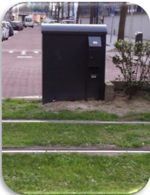
Wayside cabinet to record data from passing vehicles
